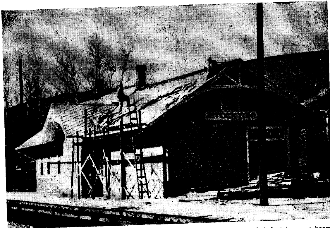
WORKMEN TEARING DOWN part of the Stockton station. It was built in an era when the mining and livestock industries were booming in the area and traffic was heavy.
